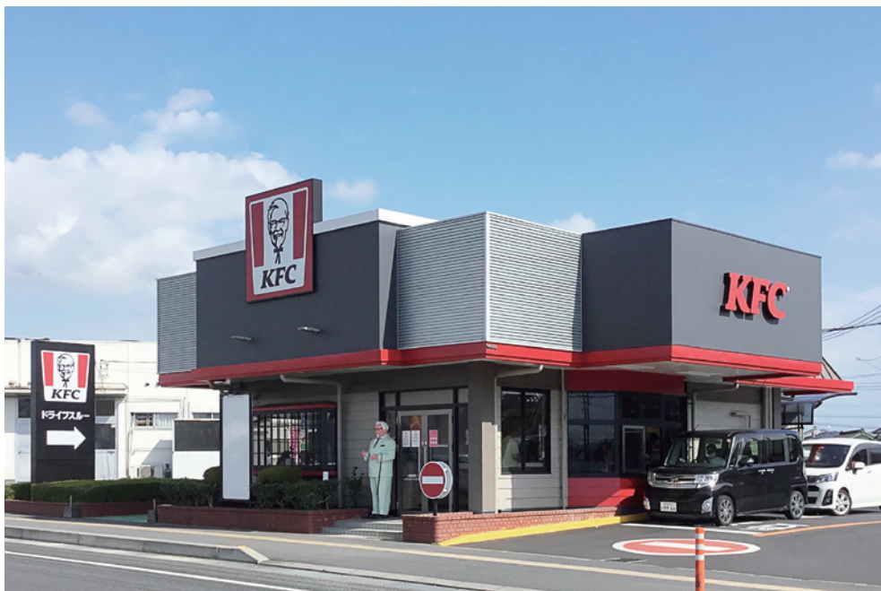
photo: KFC Kanoya (renewal)
